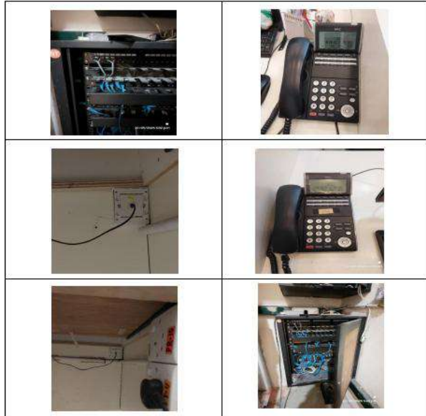
1. Cabling work (PABX) at Jakel mall Kuala Lumpur.
