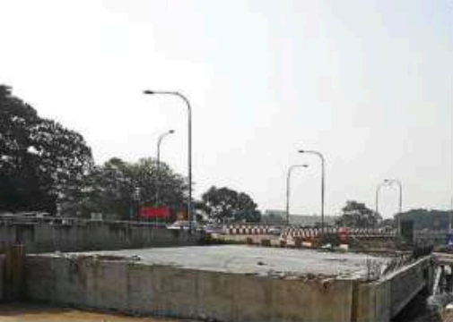
Highway construction of Middle Ring Road Seremban, Phase 3A
